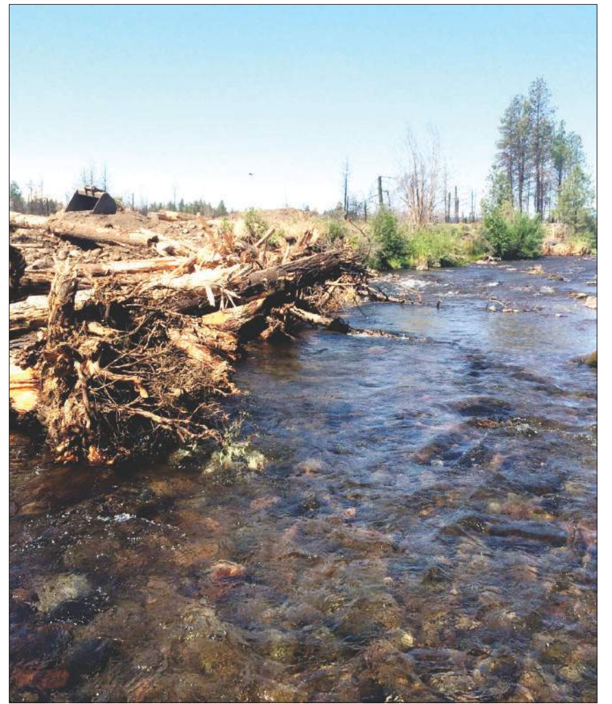
Close up of LWD Structure Downstream of B-140 Bridge
