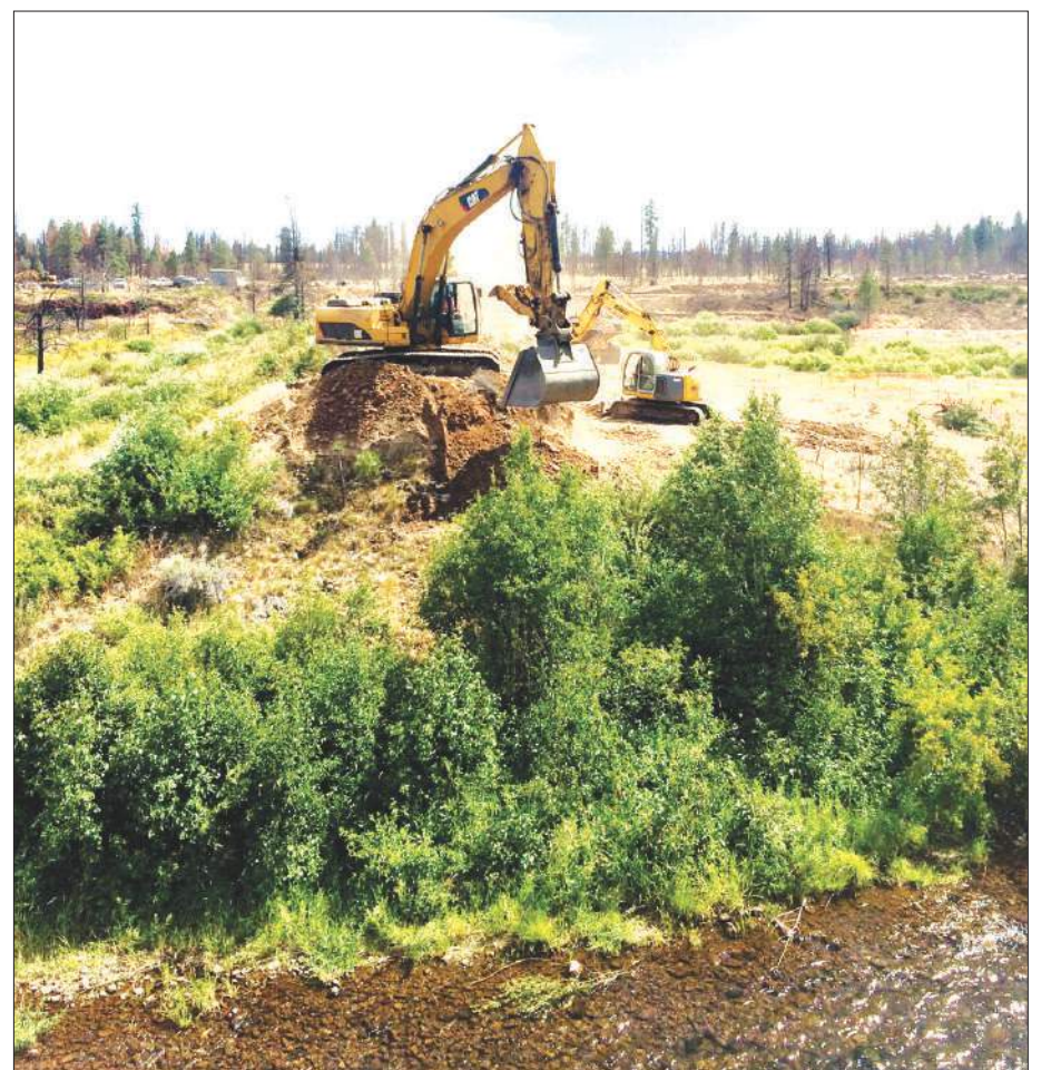
Removing the lower berm
